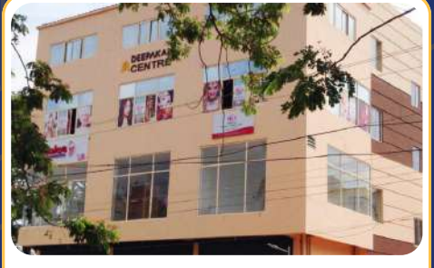
Deepakam Centre Palakkad
